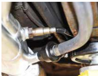
With the header installed, we added the oxygen sensor and the crankcase evacuation check valve to the collector. The fit on the driver side was excellent.
