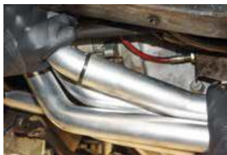
With the driver-side header installed, we slipped the cylinder No. 7 tube into place. There is no need for a clamp or gasket; the pipe slides together, and the flange at the cylinder head holds the pipe in place.
